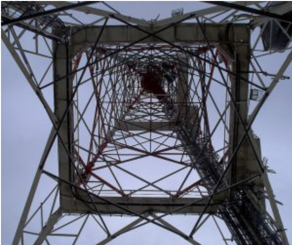
The view from below of a radio transmission tower by "Serendipiddy," CCBY. Source: Flickr.
