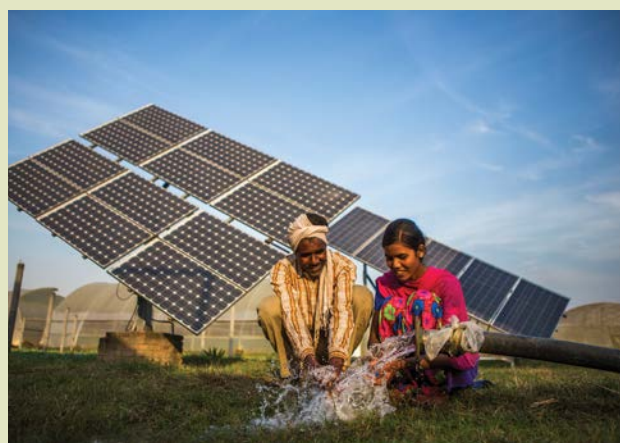
Solar pump in Jagadhri, India.
