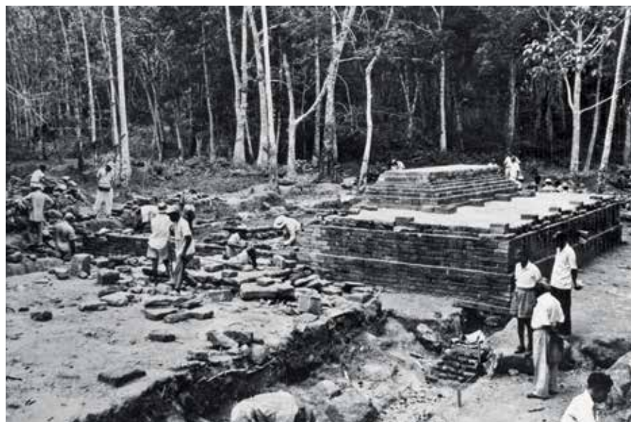
Fig. 23. Candi Bukit Batu Pahat, Bujang valley (site 8), Kedah, Malaysia. Photographed during excavation and restoration by the University of Malaya and the Malaysian Department of Archaeology in 1958–59
