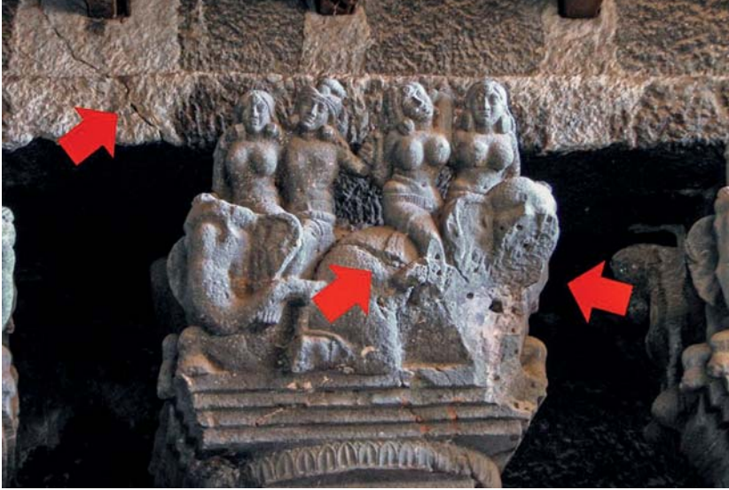
Fig. 15. Detail of flaws in the stone necessitating an ancient repair to the pillar capital. Cave 8 ( caitya hall), Kārle, 1 st century CE.
