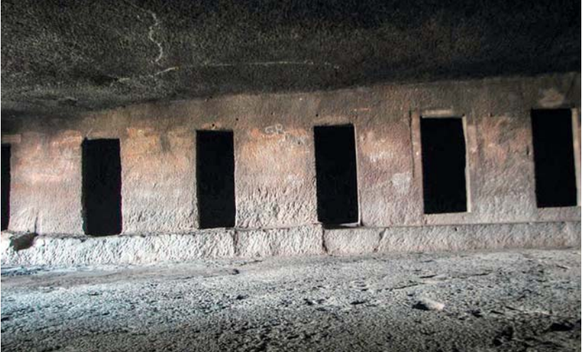
Fig. 4. Left side wall of cave. Note the rough patches on the bench towards the front (left) of the excavation. Cave 20, Nāṣik, 1 st –2 nd century CE, with additions datable to the 5 th century.
