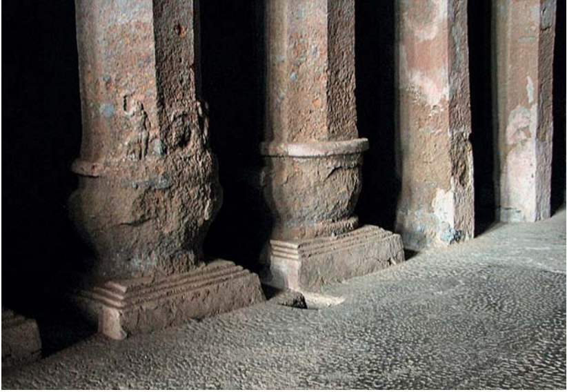
Fig. 24. Pillar bases and shafts on the left side of the hall. The fifth and sixth pillars display shafts and bases hewn from poor-quality stone (before modern restoration). Cave 3 ( caitya hall), Kānherī, 1 st –2 nd century CE.
