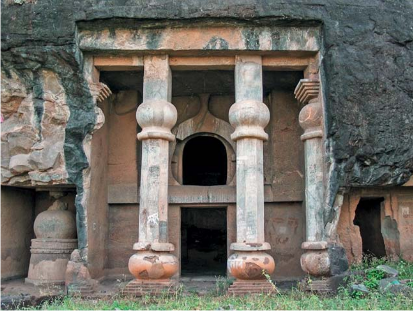
Fig. 11. Veranda with restored pillars. Cave 26, Mānmoḍī (Ambā-Ambikā), 1 st century CE.
