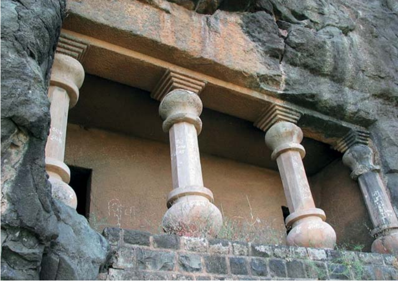
Fig. 5. Exterior view of pillared veranda. Cave 1, Mānmoḍī (Bhīmāśaṅkar), 1 st century CE.
