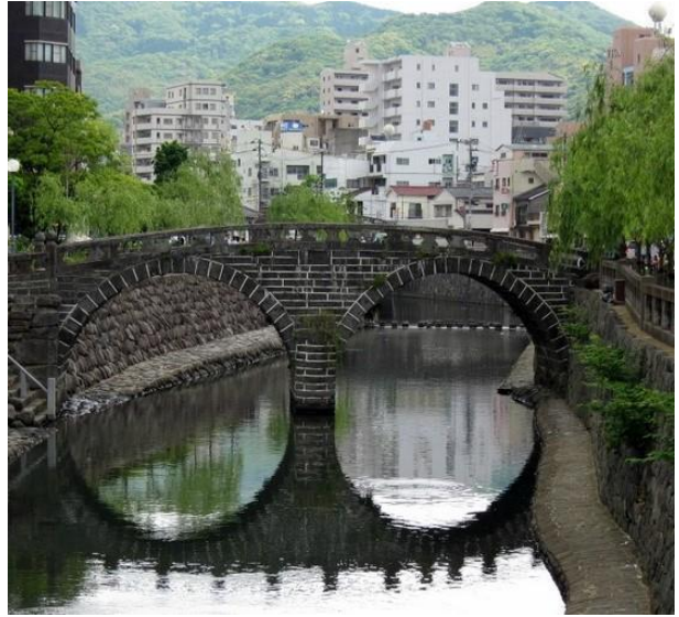
The Spectacle Bridge, Nagasaki, 1634
