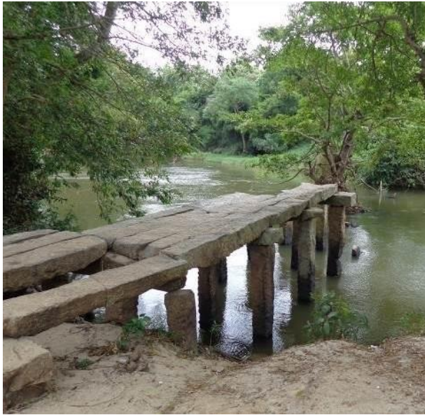
An ancient bridge in Anuradhapura, Sri Lanka
